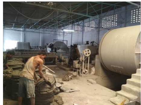
Existing ball mill
